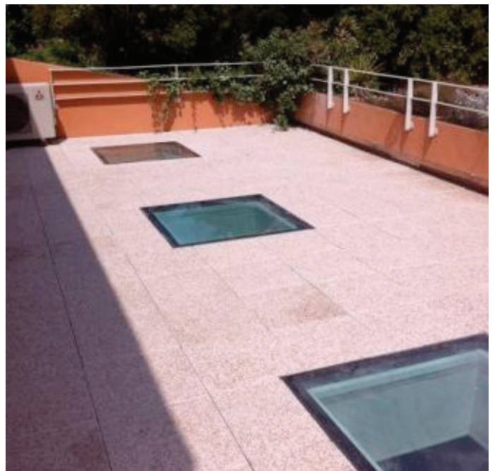
Roof terrace area
